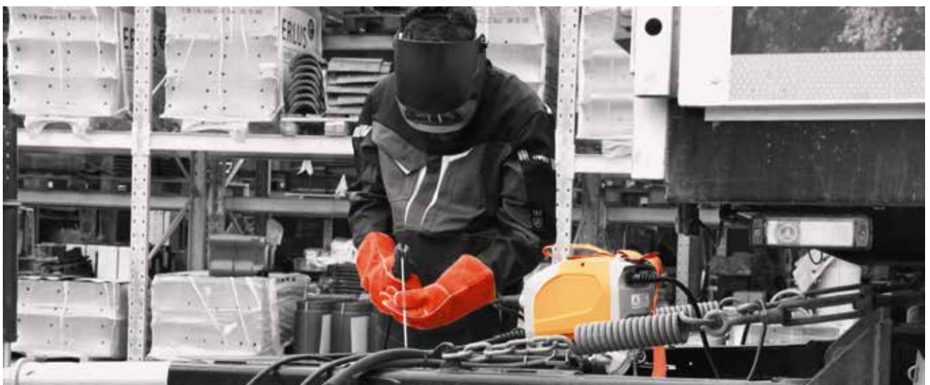
BOOSTER2 during repair work. Always reliable and ready for use.
